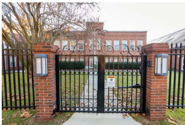
Security fencing around school buildings
