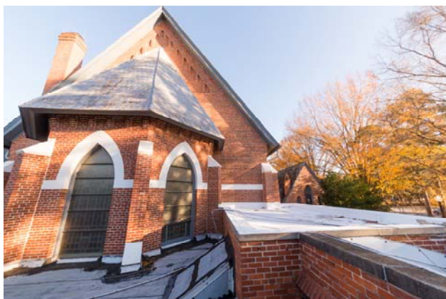
Roof repairs are underway at Old St. Mary's.
